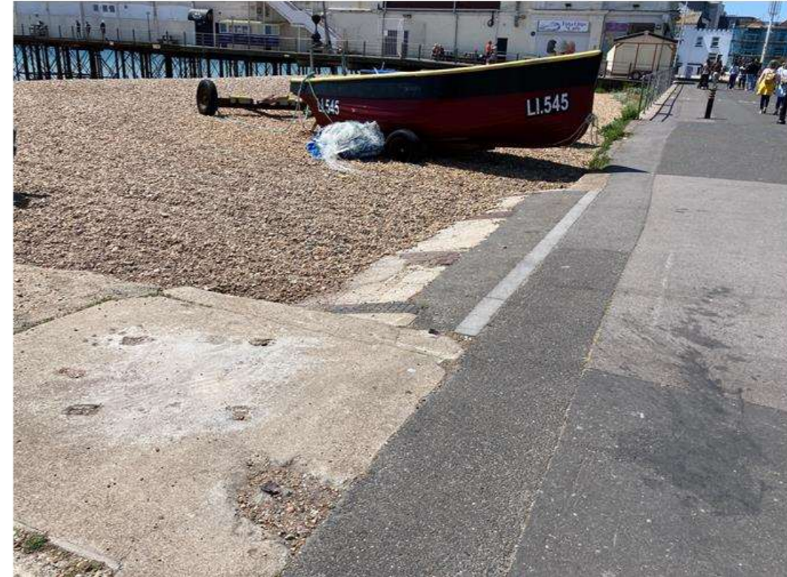
Figure 16 - Waterloo Square, May 2023
