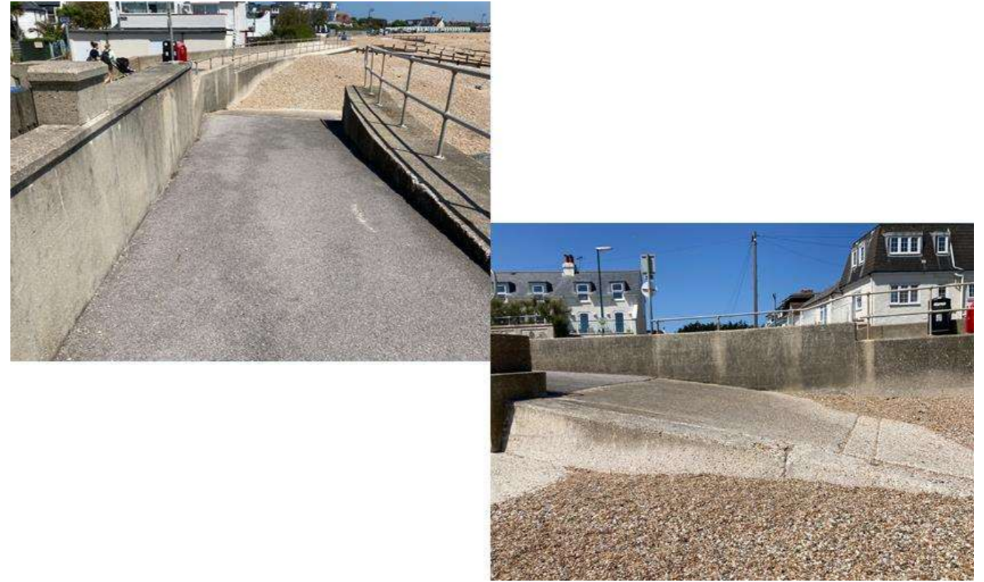
Figure 10 - Outram Road, May 2023
